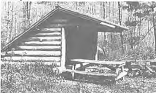
A solid, presawn and prefabricated construction was used in the Smith Shelter in Pennsylvania.
