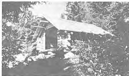
The Gentian Pond Shelter in New Hampshire was built with native logs and a shingled roof.
