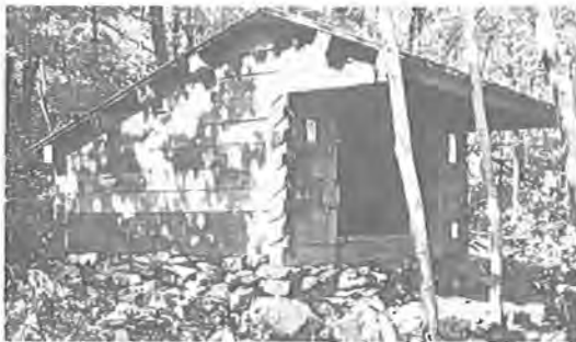
A solid, presawn and prefabricated construction was used in the Smith Shelter in Pennsylvania.
