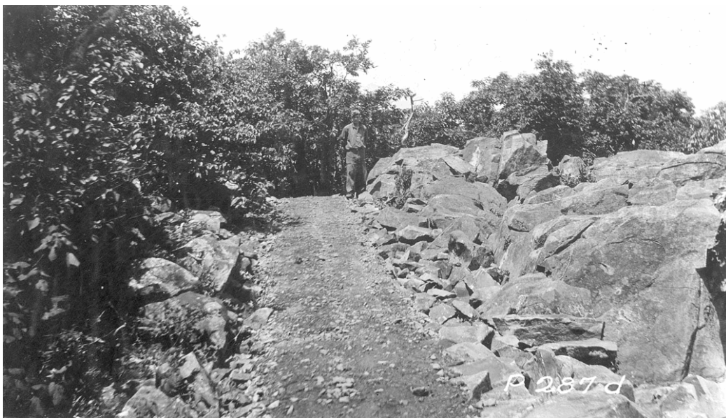
Figure 12: CCC photo showing rubble walls along AT near Mt. Marshall, circa 1935. The trail ascends at an even grade and width, with a substantial amount of gravel added for a durable tread. (Shenandoah NP Archives)
