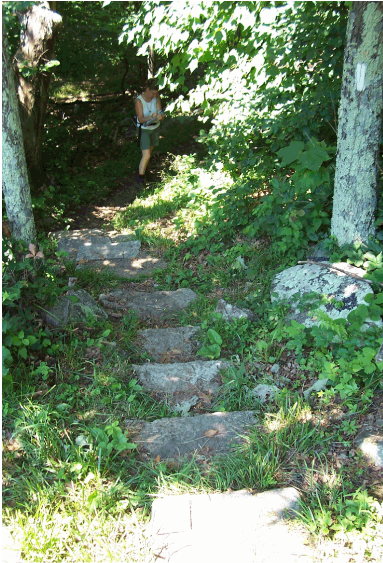
Figure 23: Slab-laid stone steps, built by the CCC in the 1930s near the north end of Hogback Overlook. The CCC stonework was often built in association with overlooks to accommodate a wider range of hiking abilities. (SUNY, 2006)
