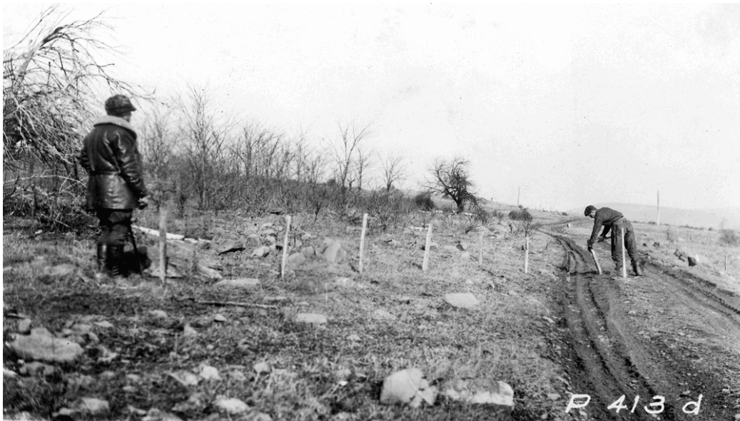
Figure 4: Civilian Conservation Corps (CCC) photo showing two men staking the alignment of the AT near Range View Cabin, circa 1935. (Shenandoah NP Archives)
