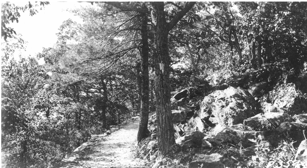
Figure 8: CCC photo showing completed Neighbor Mountain side trail, circa 1935. The trail has a width of 42-48 inches, is edged with stones, and is surfaced with gravel. (Shenandoah NP Archives)
