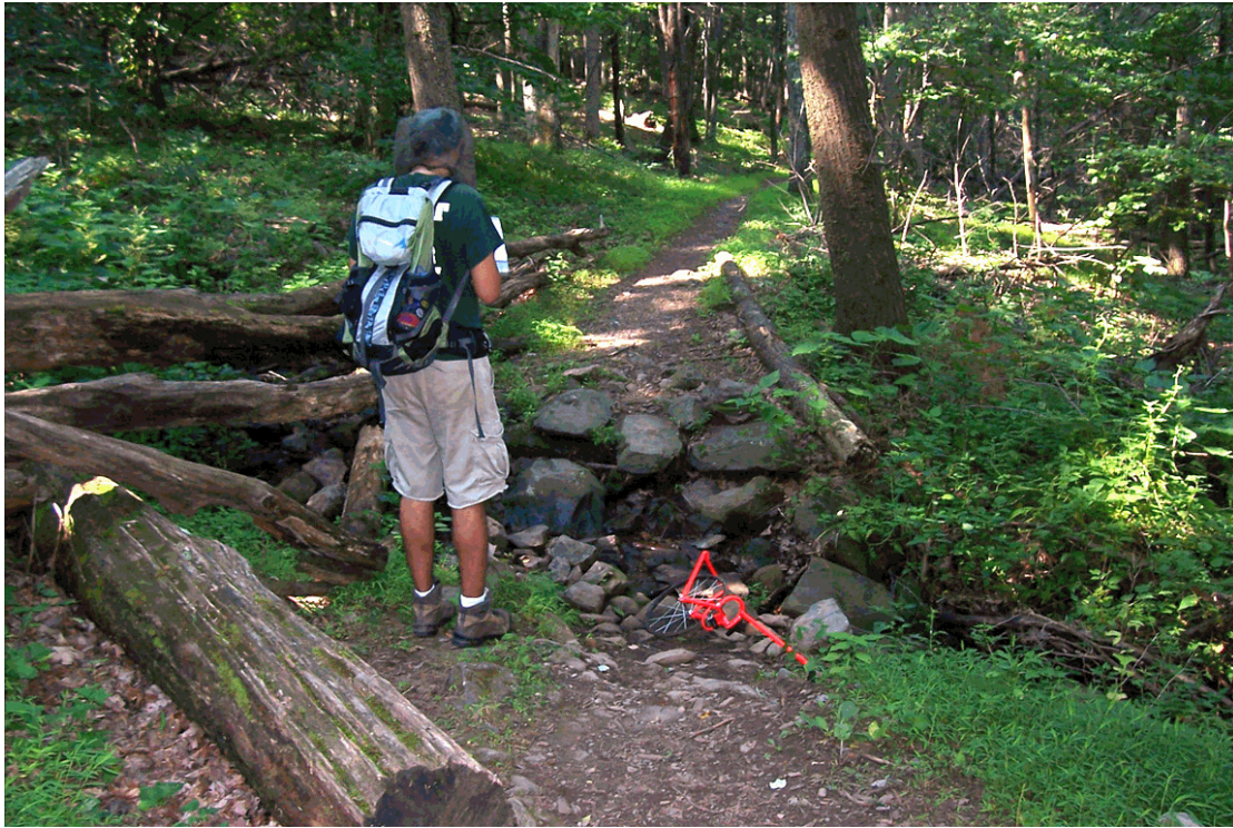
Figure 15: The AT crosses a stream near Elkwallow Gap. A collapsed abutment suggests the CCC may have constructed a small bridge over the stream to provide an even walking tread. (SUNY, 2006)
