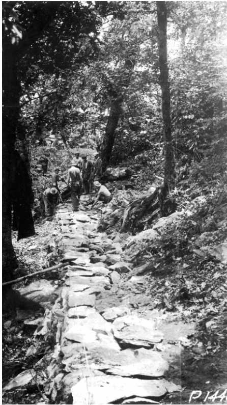
Figure 5: A CCC crew constructing a retaining wall for the AT, which will be surfaced with a gravel walking tread, circa 1935. A string line is used to guide stone placement (location of photo unknown). (Shenandoah NP Archives)
