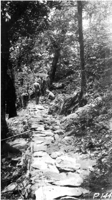
Figure 12: A CCC crew constructing a retaining wall for the AT, which will be surfaced with a gravel walking tread, circa 1935. A string line is used to guide stone placement (location of photograph unknown). (Shenandoah NP Archives)
