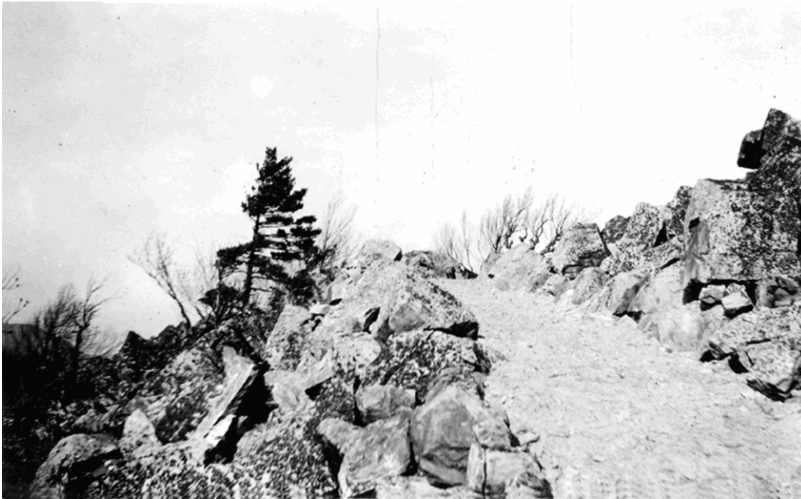
Figure 6: CCC photo showing the completed section of trail along Blackrock, circa 1936. The treadway is evenly graded and surfaced with gravel. The trail width is 42-48 inches with a 3 percent cross pitch. (Shenandoah NP Archives)
