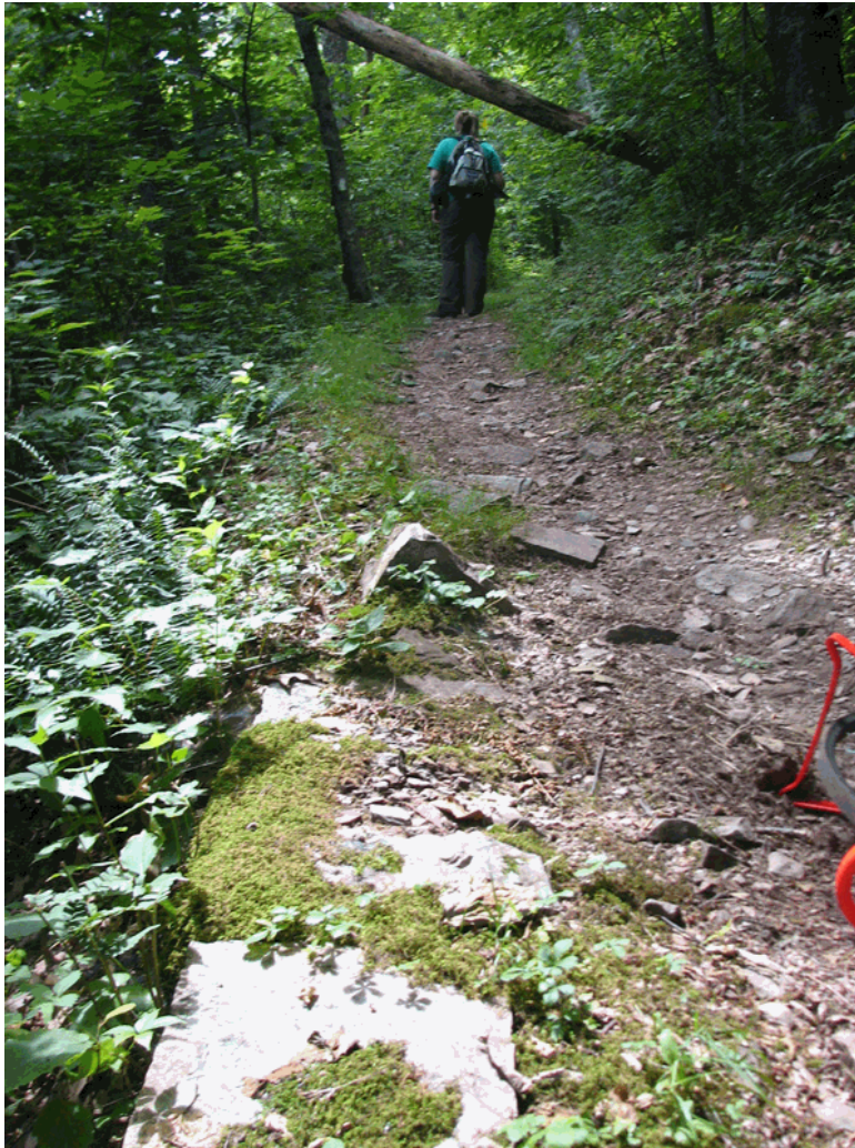
Figure 19: The CCC-graded trail has eroded, forming a slight gully in the middle of the trail and has not retained the three-percent cross pitch. (SUNY, 2006)
