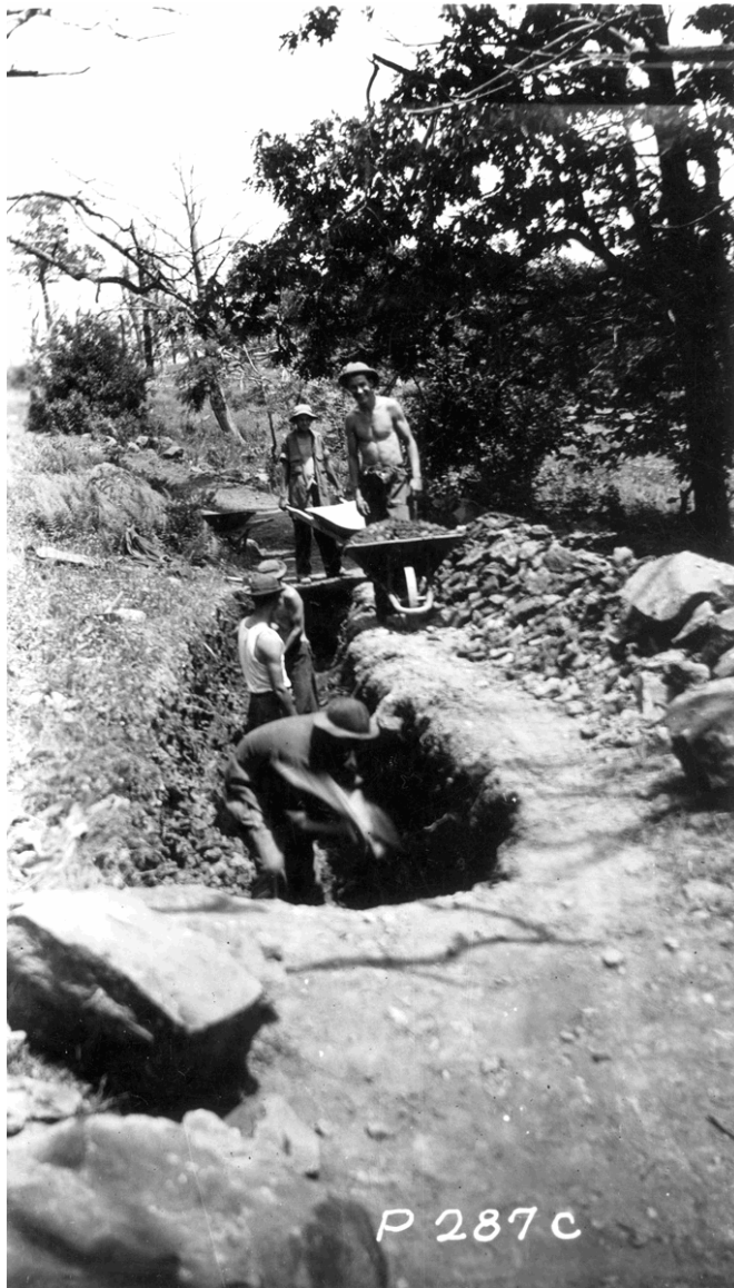
Figure 4: A Civilian Conservation Corps (CCC) photo showing men digging shale for trail construction near Loft Mountain, circa 1935. (Shenandoah NP Archives)
