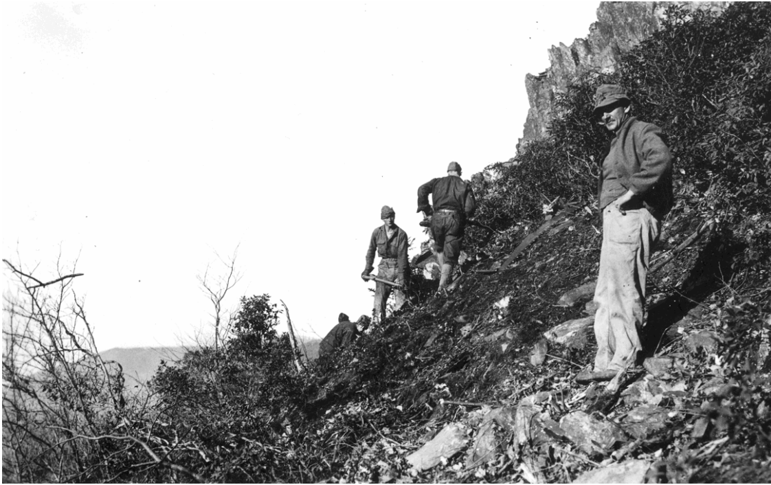
Figure 4: Civilian Conservation Corps (CCC) photo shows men conducting preliminary work on the AT south of Crescent Rock. The trail bed was built out from the steep slope to support the trail circa 1935. (Shenandoah NP Archives)
