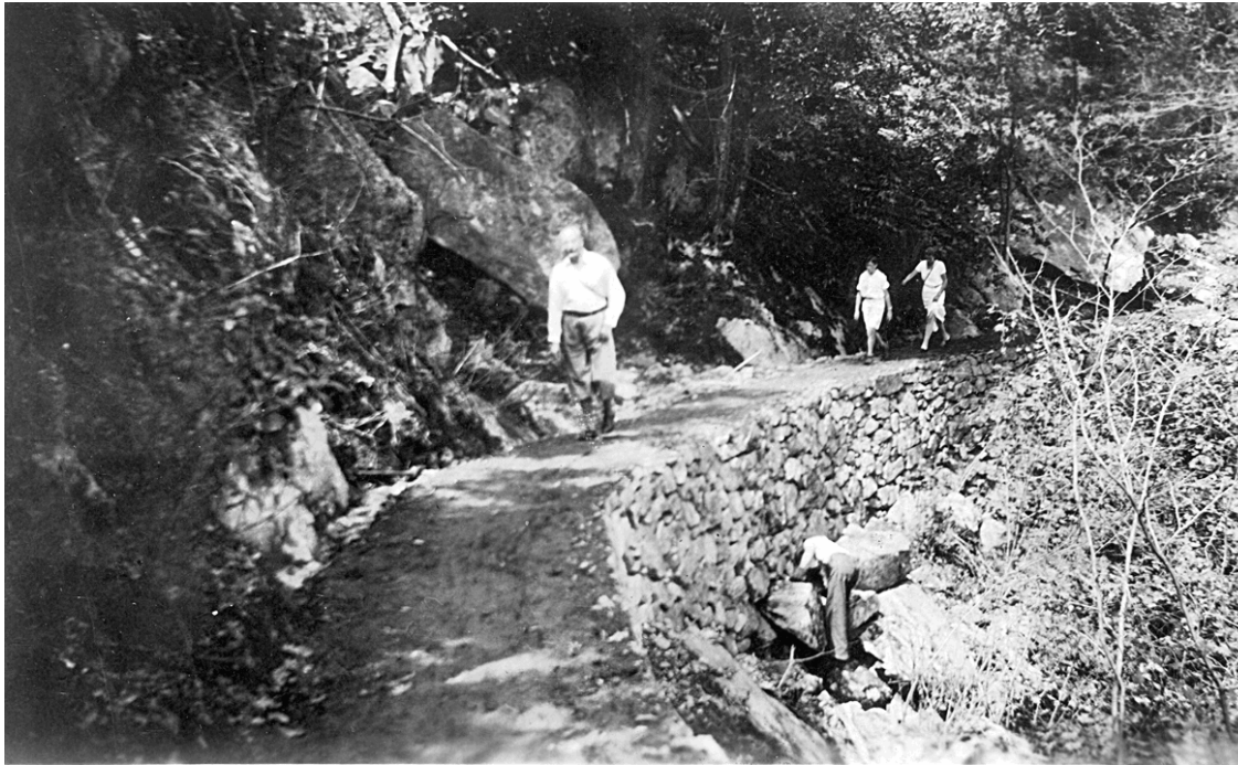
Figure 11: CCC photo showing the AT to Mary's Rock, circa 1935, and a large stone retaining that supports a trail bed built out from the steep slope. Both the trail and wall display a graceful sweeping curve. (Shenandoah NP Archives)
